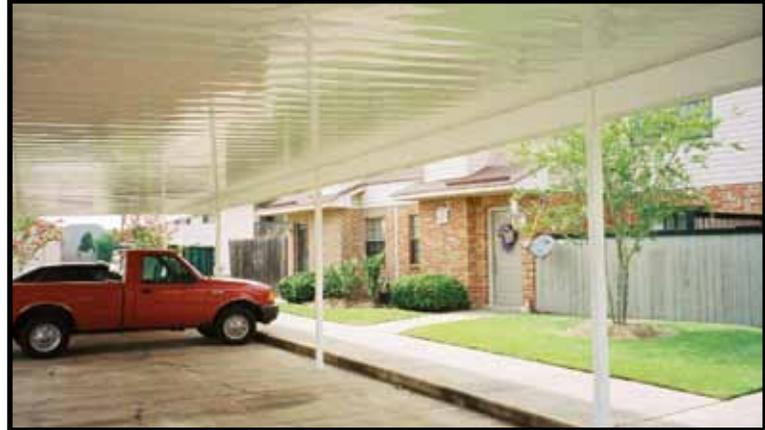
*Below: This gabled walkcover constructed of roll-formed pan is structurally more sound, drains better, and offers an aesthetically interesting walkcover.*
